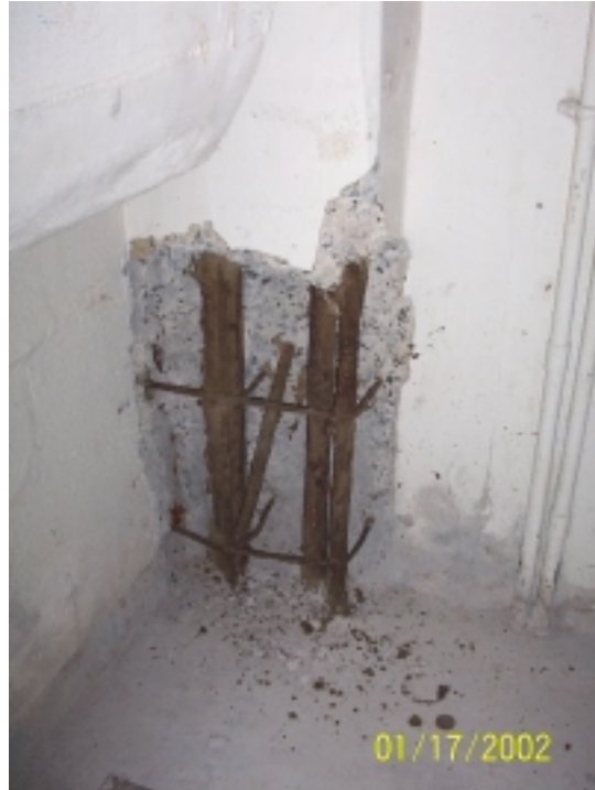
Reinforcing Corrosion
